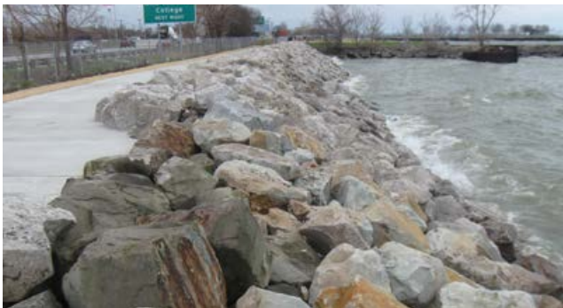
Image 7-6: Revetment Rehabilitation
