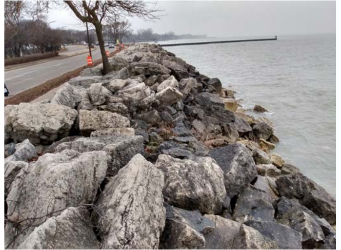
Image 2: Widening crest protection moving north
