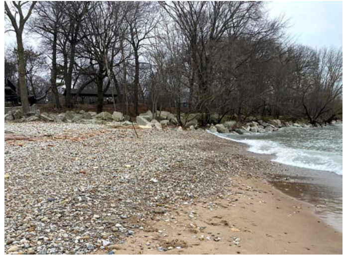
Image 2: Significant stone buildup and beach narrowing
