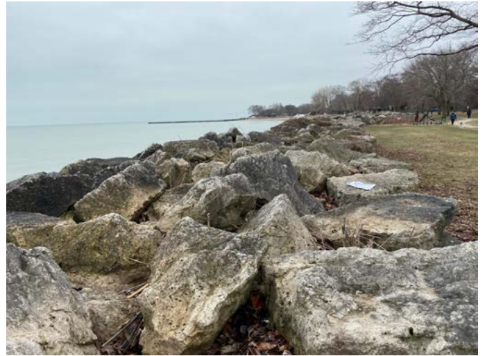
Image 2: Widening revetment crest
