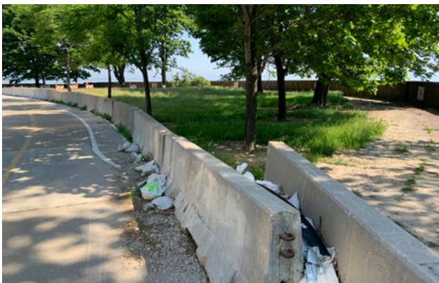
Image 7-2 Temporary Concrete barriers at 67th Street, Chicago
