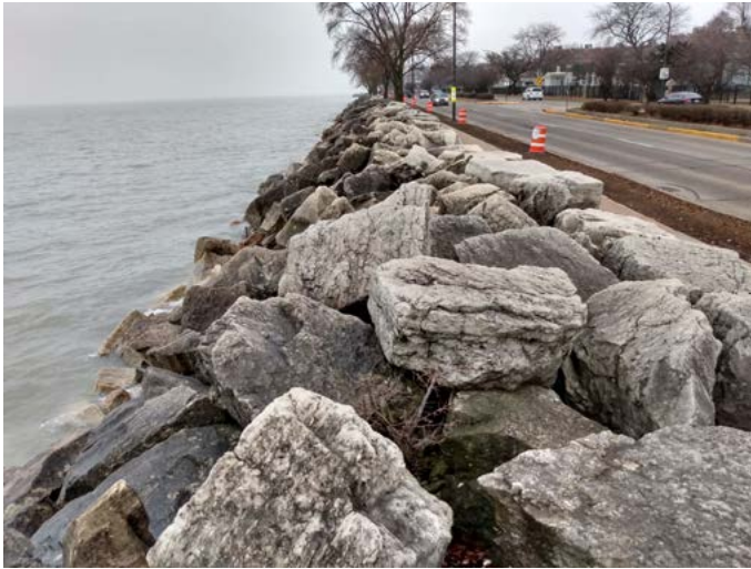
Image 1: Varying revetment slope
