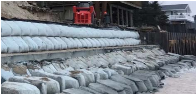
Image 7-5: Trapbag - Concrete Filled
