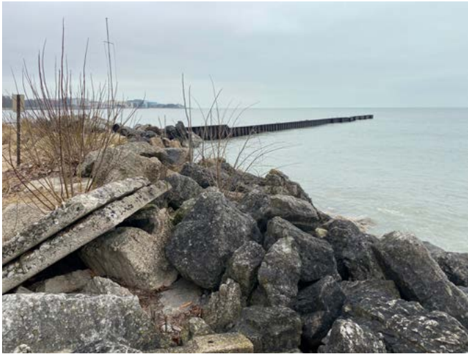
Image 1: Steep revetment slope
