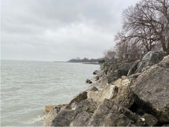
Image 1: Revetment stone stacked at near vertical slope
