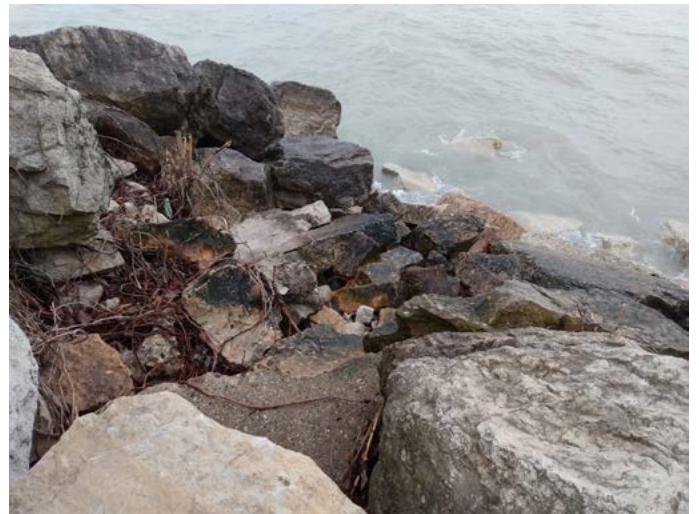
Image 4: Varying stone sizes along revetment slope
